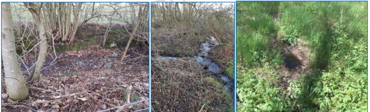
Photo 7 (left) Ponded water in agricultural drainage ditch at NW border of SE Unit; Photo 8 (right) confluence of the tributary of Shadow Brook and the drainage ditch within the alder woodland; Photo 9. Furrows and depressions saturated with water following rainfall in meadow field of SE Unit.
